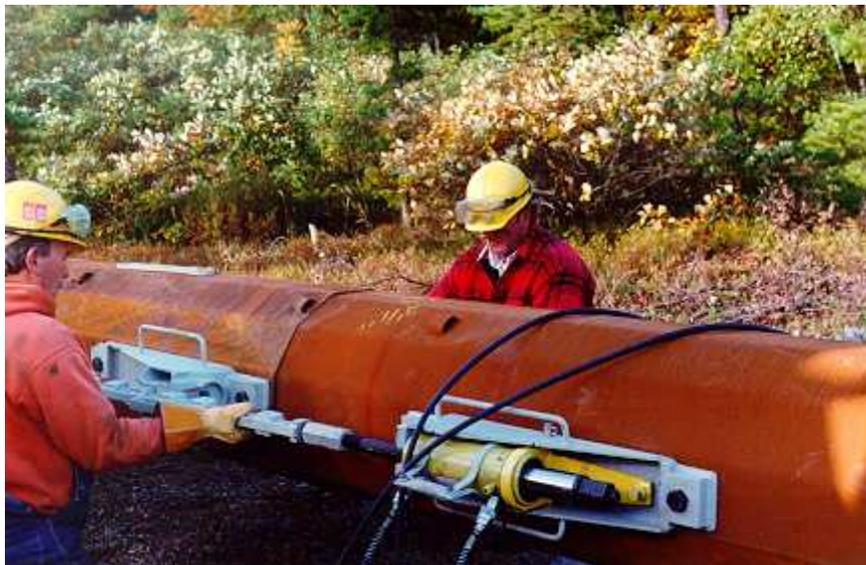
***Attaching rams with the ratchet extensions to the jack frames.***
