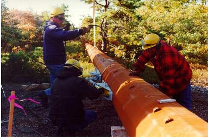
***Align pole sections, then attach jack frames to both sides of each shaft section using the 1" diameter bolts.***
