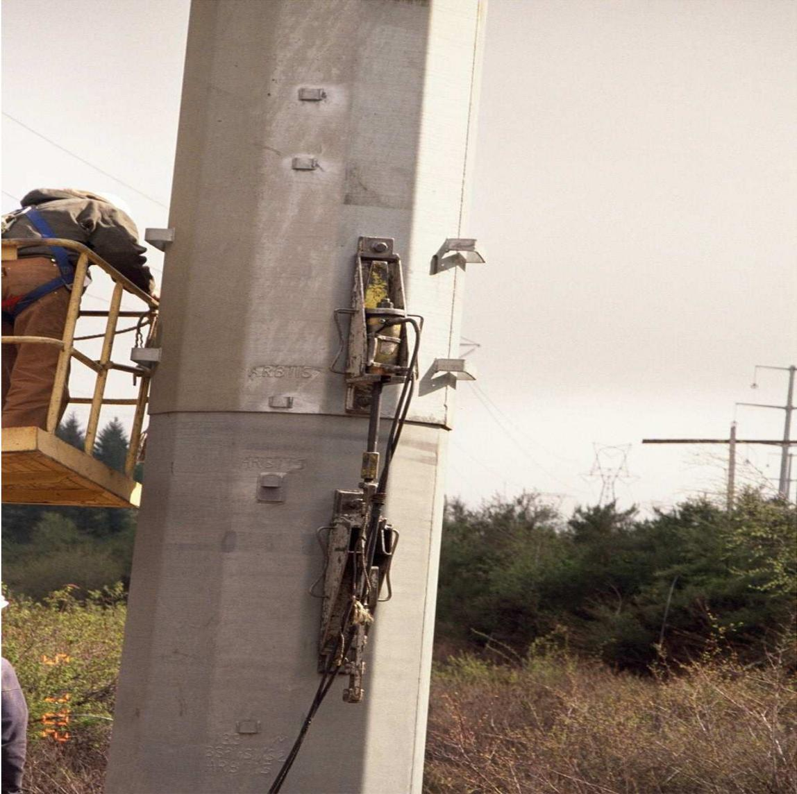
The same basic methods for assembly of slipjoints is applicable to structures that are erected in sections. Normally, the weight of the upper section does not exceed the design force and jacking is still required. The jacking units can be mounted/operated in the vertical position. In cases when embedded stubs are set prior to the installation of the top section, special attention to the orientation/plumbness of the stub section is required.
