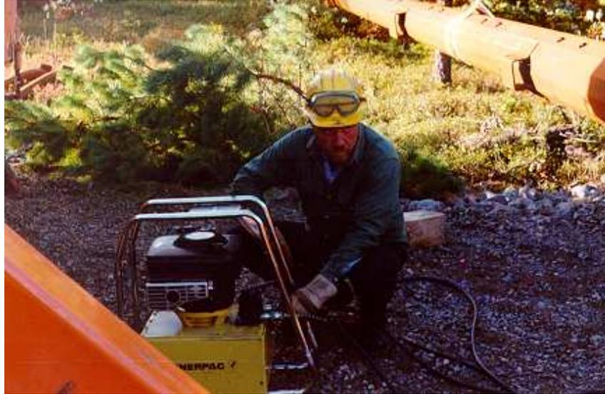
*Attaching hydraulics from the jacks to the Enerpac unit.*
